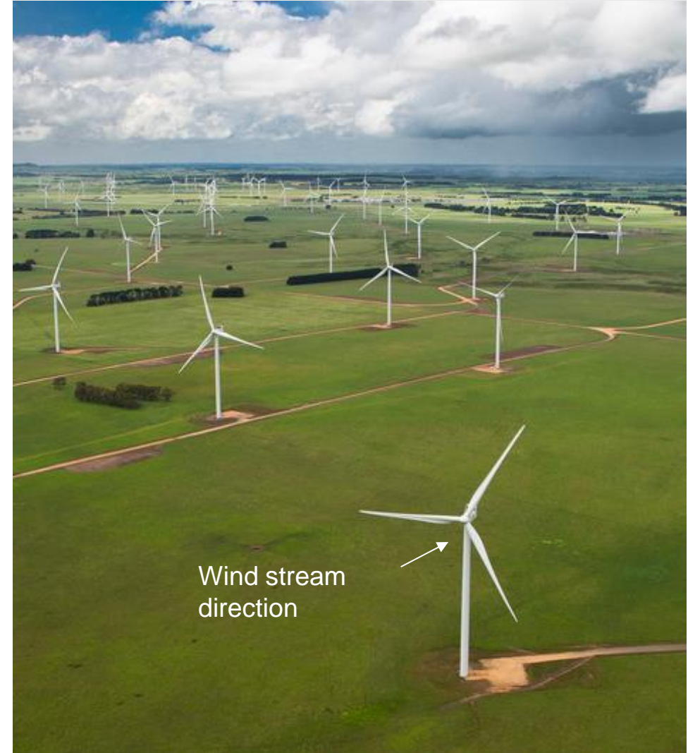
Macarthur Wind Farm, Australia
